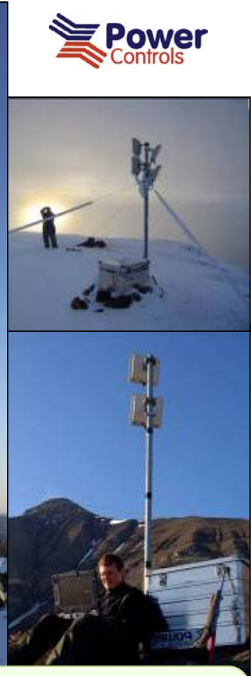
Repeater Stations EFOY Pro in Insulated Outdoor Box (Norway)
