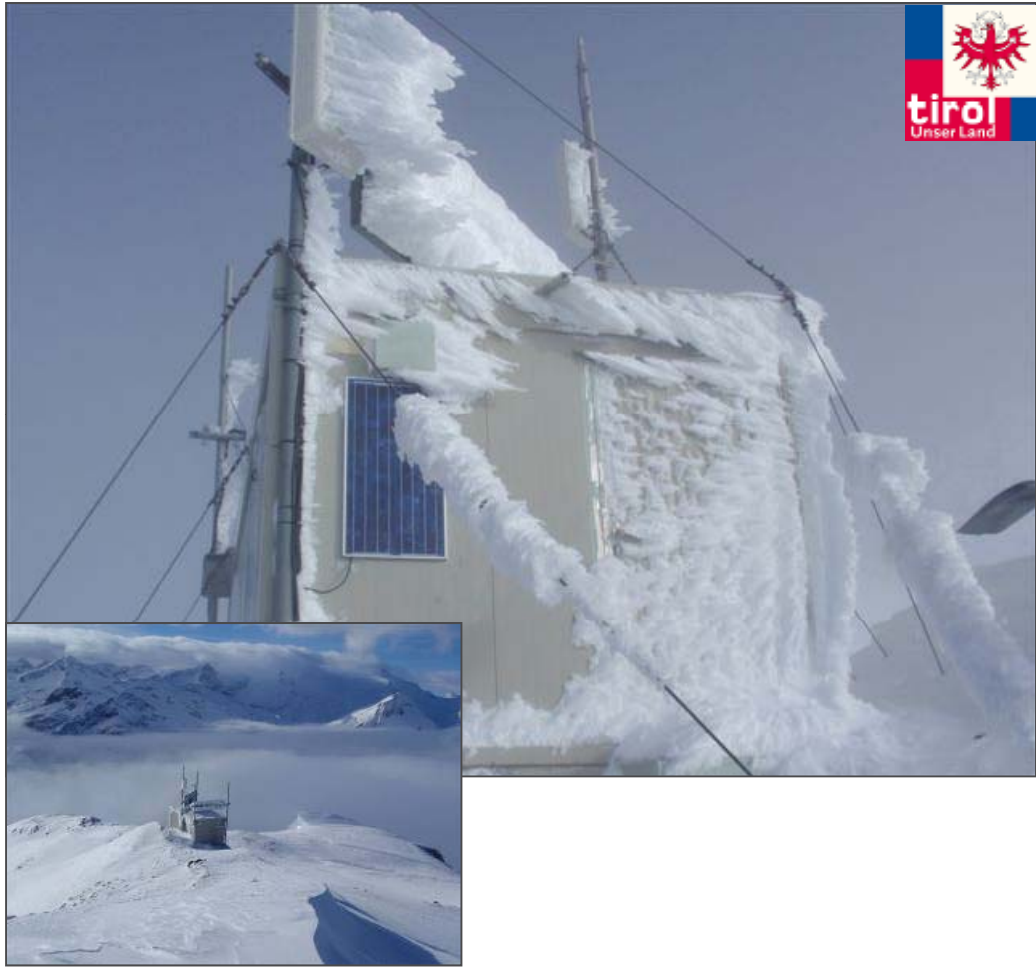
Base Transceiver Station (Austria) with 4 EFOY Pro 1600
