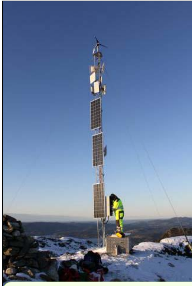
Repeater Stations EFOY Pro in Insulated Outdoor Box (Norway)
