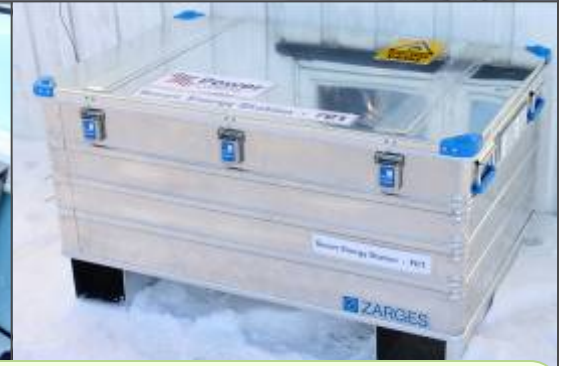
Internet via Radio Link Mast, EFOY Pro in Insulated Outdoor Box (Norway)
