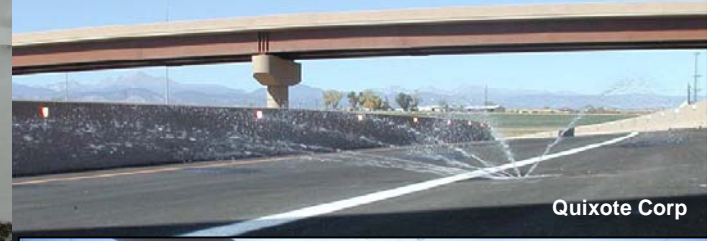
Fixed Anti-Icing Spray Technology (FAST)
