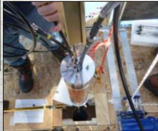
Antenna being deployed into hole
