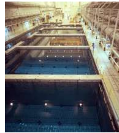
Fuel and Storage Facility
