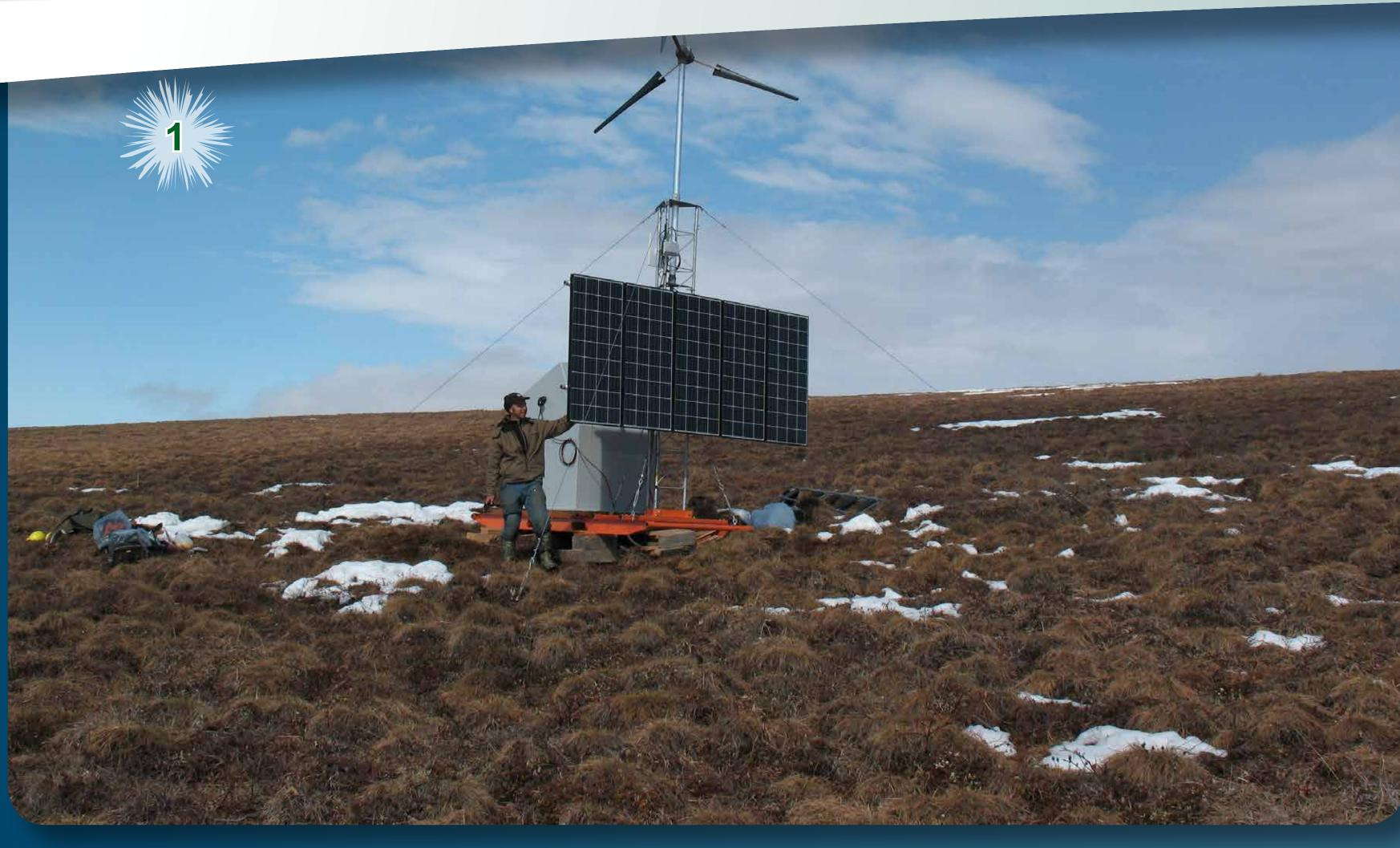
1. Imnavait Creek, Alaska. Autonomous year-round hybrid solar / wind power system with conventional south facing 650 Watt PV array. Steep angle sheds snow and maximizes winter solar production. This system was designed by ABS-Alaskan, deployed and maintained by CH2M HILL Polar Services.
