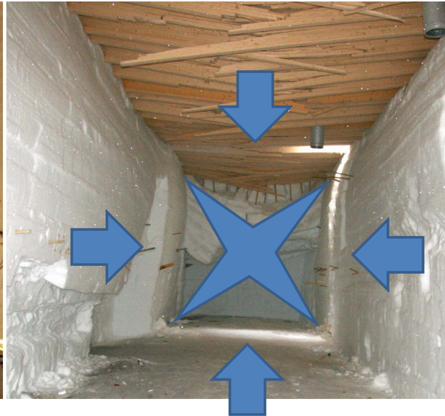
Compressive slumping dynamic of all four surfaces
